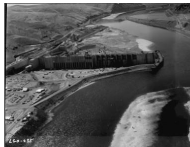
Image A. Lower Granite Dam year 1970.
