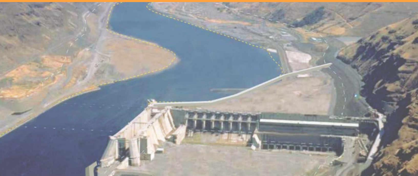
ABOVE PHOTO SIMULATION OF A LOWER GRANITE CHANNEL BY-PASS WRITTEN IN THE 2002 EIS
