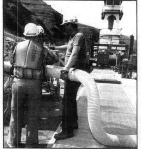
Plastic pipe transports juvenile fish from dam bypass system into fish transportation barge.
