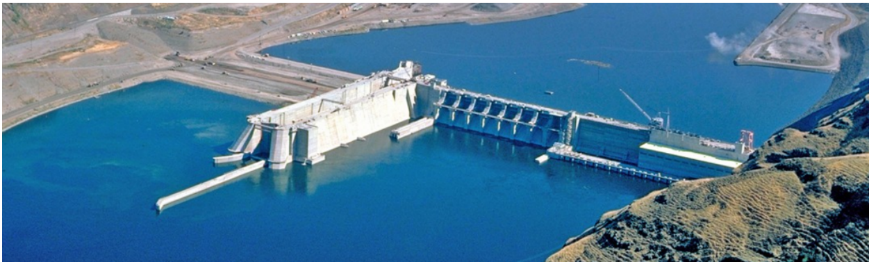
Lower Granite Dam during embankment construction photo. Embankment removal would look similar.
