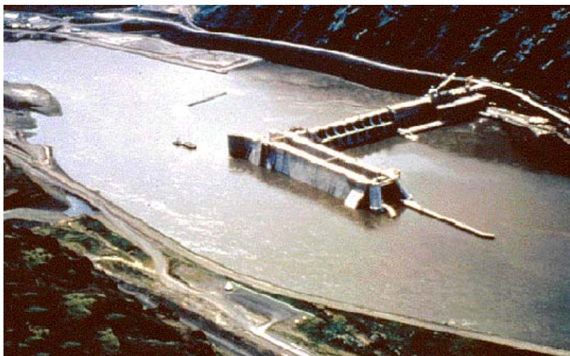
Photo of Lower Granite Dam taken during dam construction. The channel existed in this configuration for several years.
