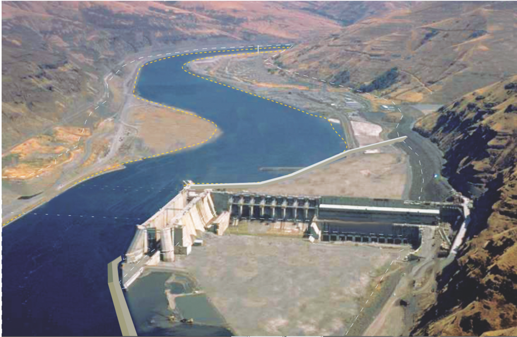
Lower Granite Dam with Channel Bypass
