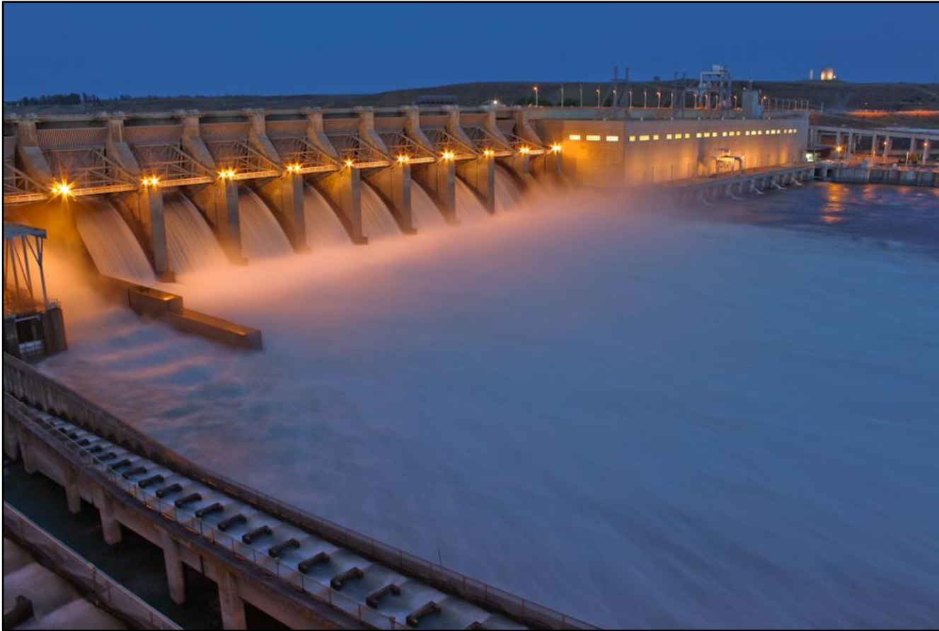
Ice Harbor Dam
